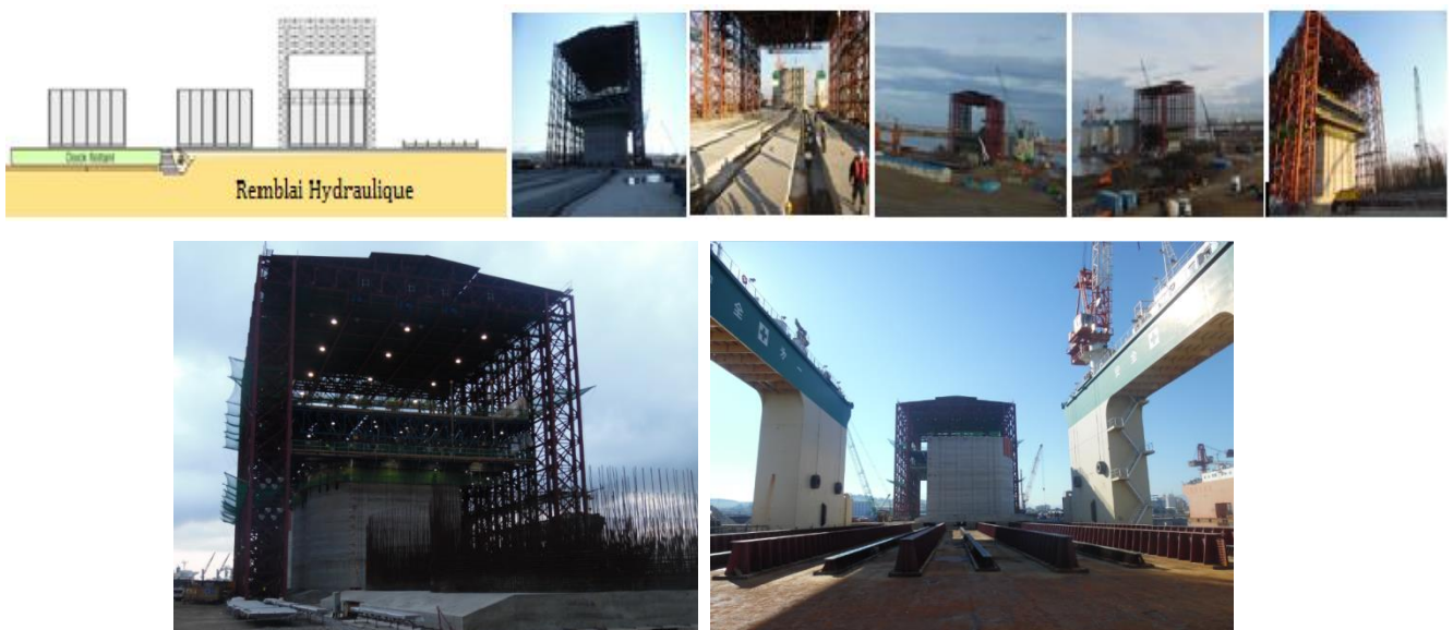
Figure IV. 13: (a) Caisson manufacturing workshop [57].
