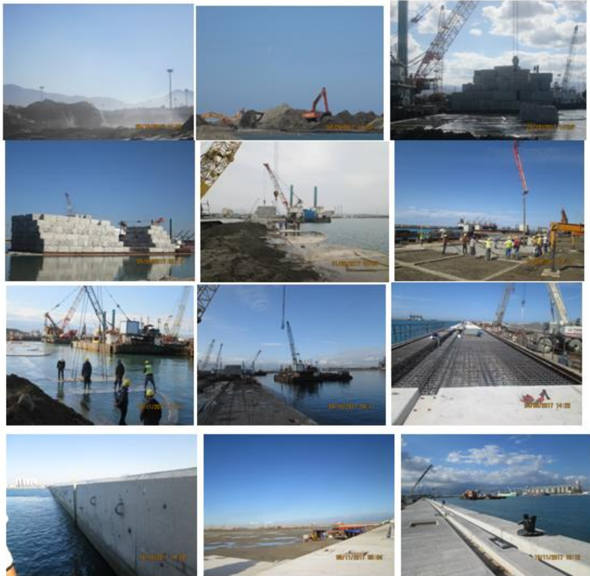
Figure V. 11: Photography's of quay wall works [56].
