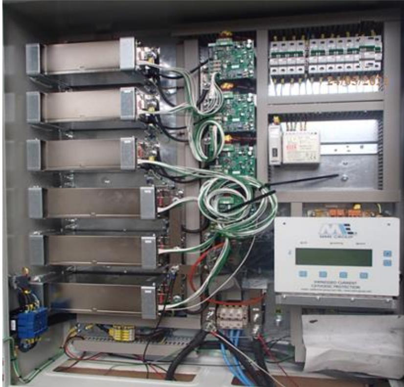
Fig. 5.8: The prototype ICCP of the measuring and control box
