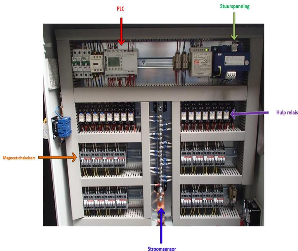
Fig. 4.20: Front side of the variable load resistor
