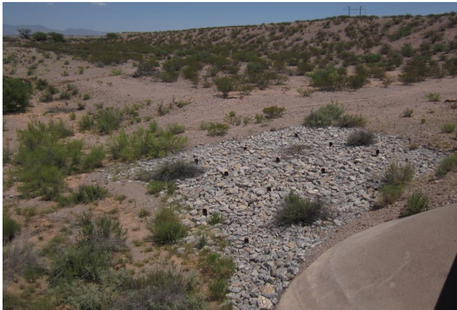
Figure 32: Engineered conveyance system using riprap.
