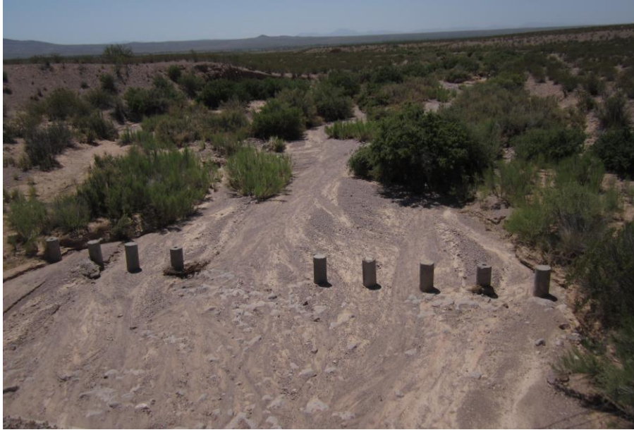
Figure 31: Geoengineered erosion control system to reduce stormwater flow velocity.
