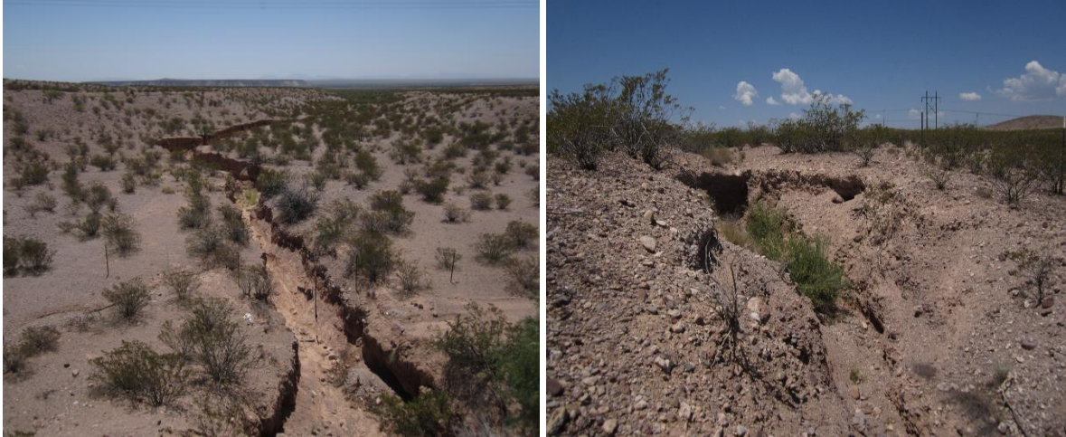
Figure 13: Evidence of erosion and mass movement of materials near sampling location.
