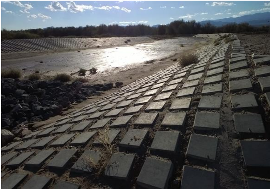
Figure 30: Hard armor erosion control system.
