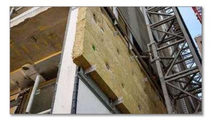
Pic. 3.9: Rockwool insulation in walls and slab (<u>Ref 3.10)</u>
