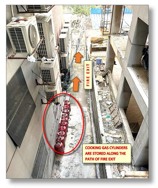
*Pic. 5.1.9*: Fire safety is at stake in this scenario The orange arrow shows the escape way direction from the fire stair (Ref: Self-sourced, 2024)
