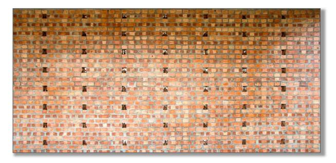
Pic 4.43: Karupannya-rangpur-factory's wall made of clay brick woth perforation to allow wind
