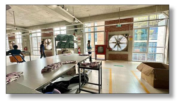
Pic 5.4.19: Exhaust fan installed in the working areas to keep the area cool (Ref:ss)
