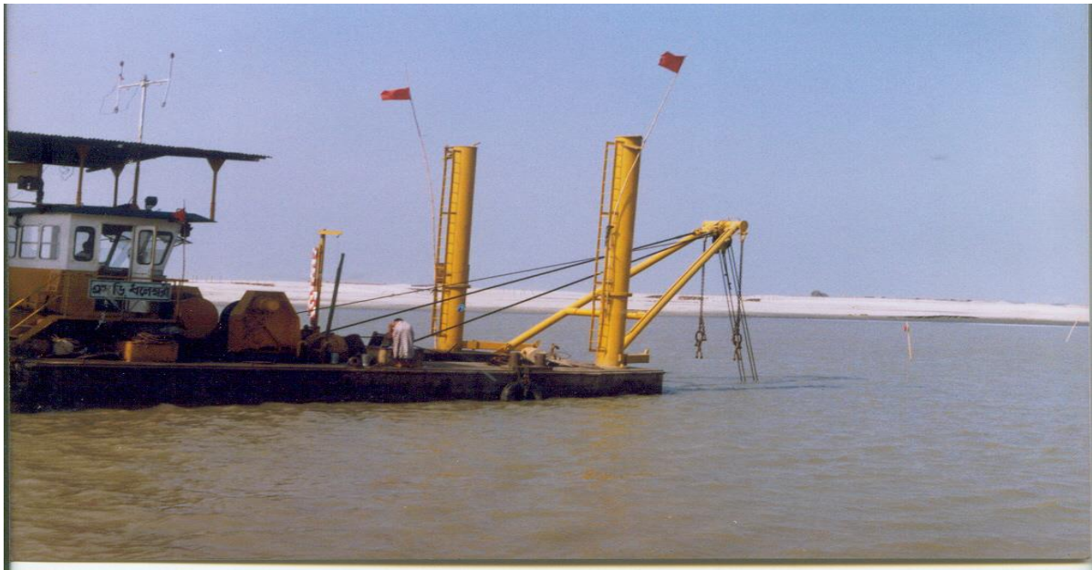
Figure 1-4: Dredger D-136 - CSD of BIWTA is in action in the Meghna River
