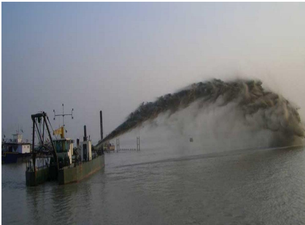
Photograph 3-2: River dredging – Open discharge (source BIWTA)
