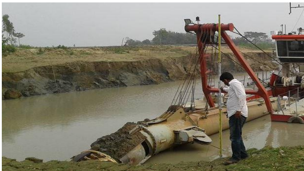
Photograph 3-4: 155-km-long Bhogai-Kangsha river route dredging works in Netrokona (Source BIWTA)
