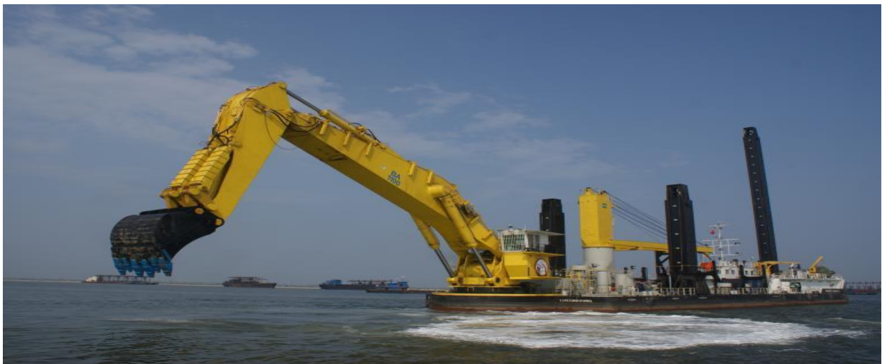
Figure 2-6: Backhoe dredger in action
