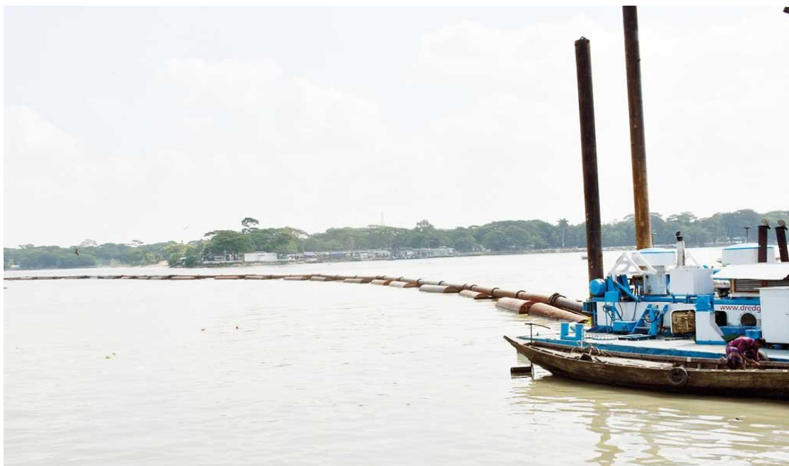
Photograph 3-3: Dredging surrounding Barishal Inland River Port areas to ease the navigability crisis for river transportation in Barishal region (Source: Dhaka Tribune)
